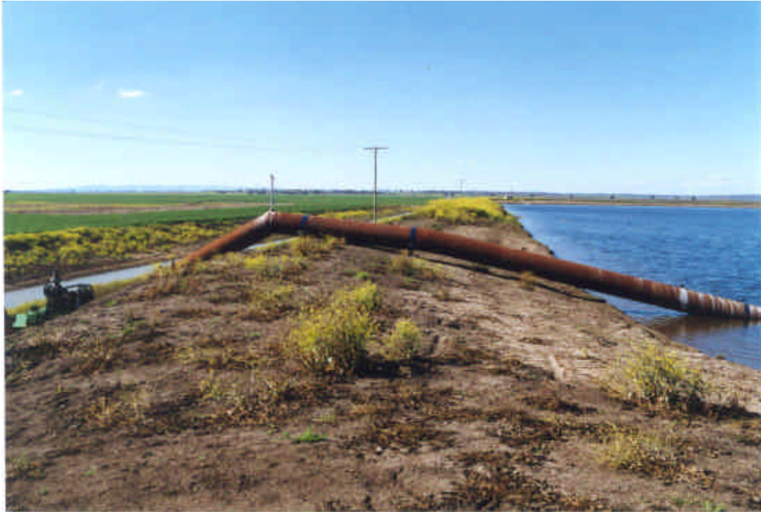
PHOTOGRAPH 5-8 – PIPELINE OVER THE EMBANKMENT
