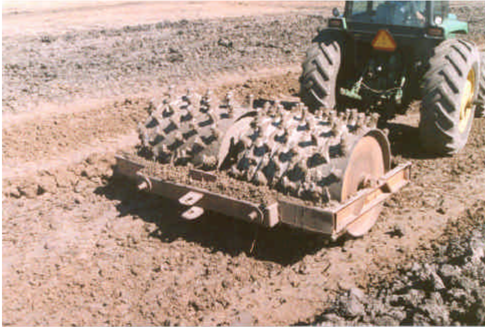
PHOTOGRAPH 5-4 – COMPACTION OF CUT-OFF TRENCH WITH ROLLER
