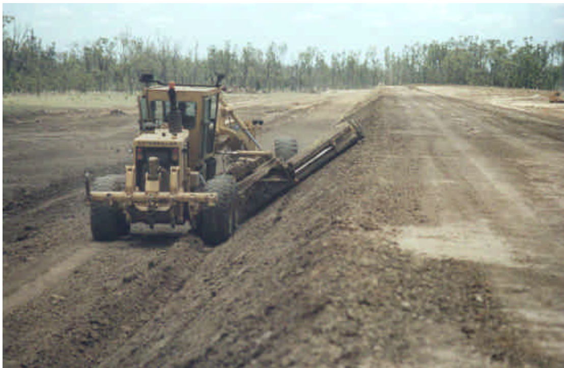
PHOTOGRAPH 5-6 – GRADER TRIMMING EMBANKMENT
