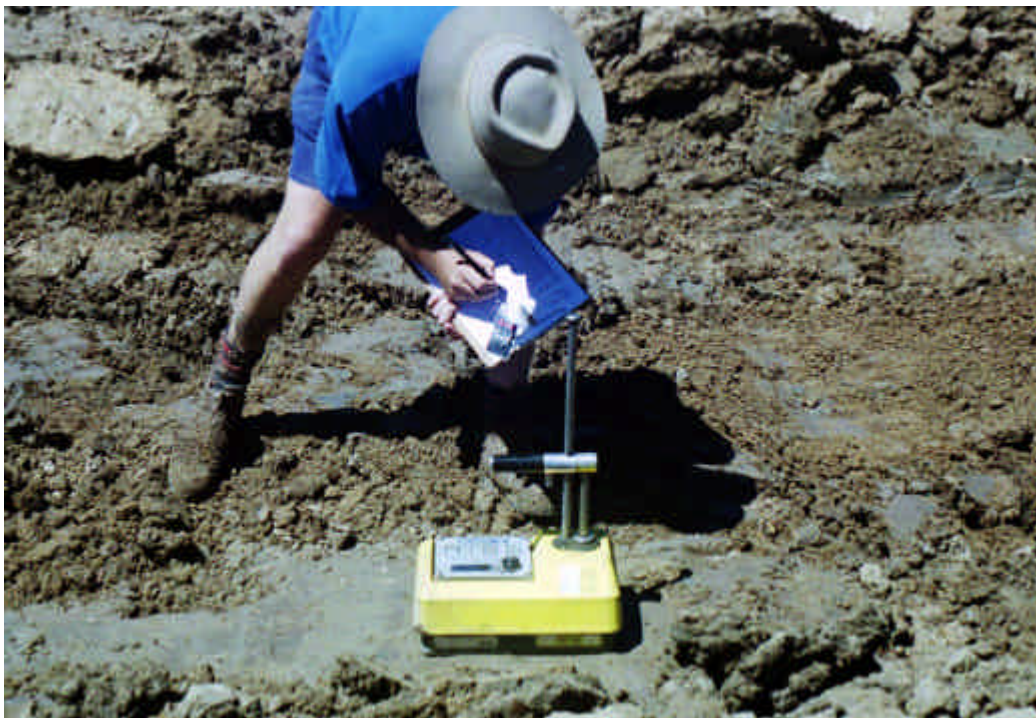
PHOTOGRAPH 5-5 – COMPACTION TESTING USING A DENSOMETER
