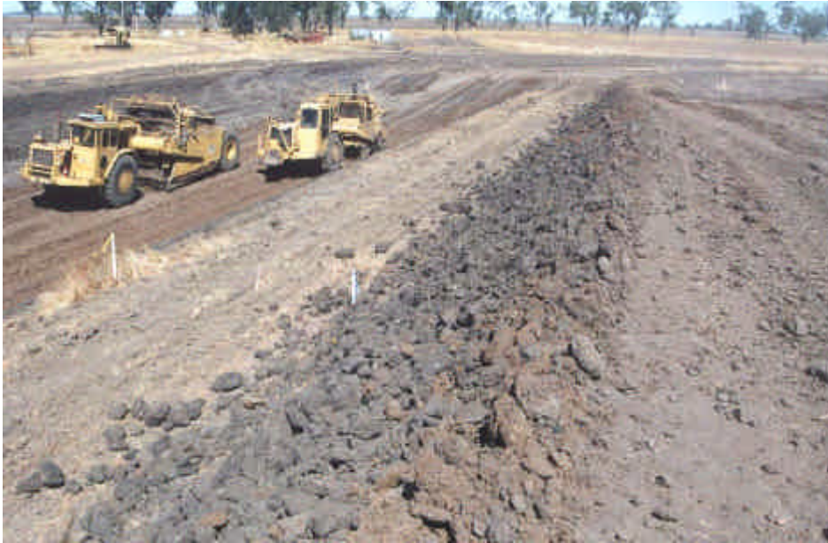
PHOTOGRAPH 5-1 – ELEVATING SCRAPERS IN BORROW PIT
