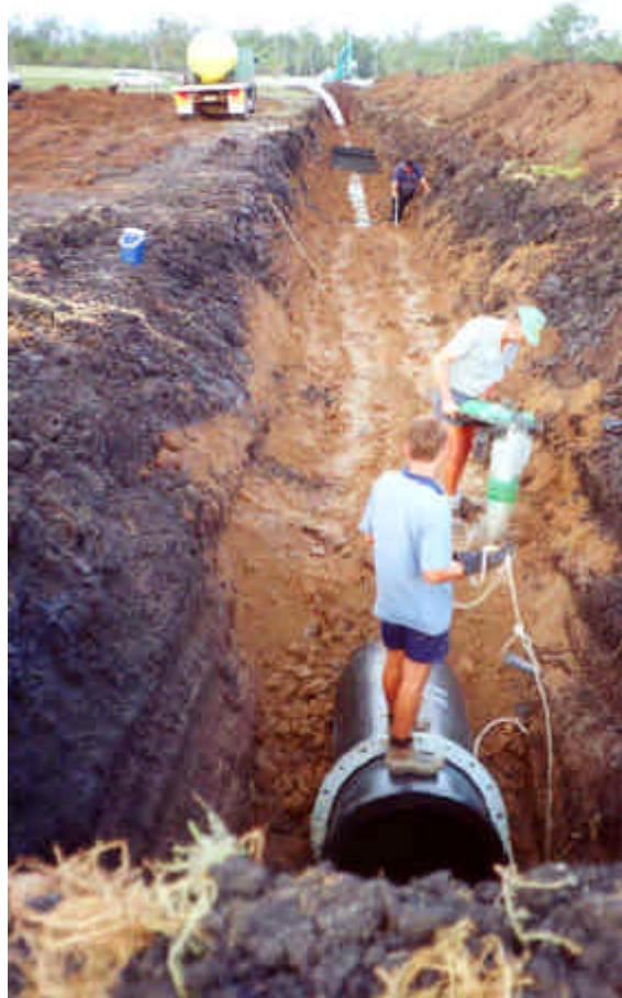
PHOTOGRAPH 5-9 – INSTALLATION OF PIPELINE UNDER EMBANKMENT
