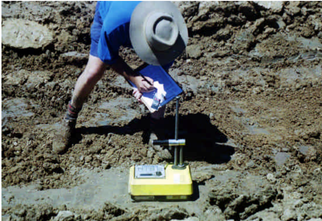
PHOTOGRAPH E-5 – UNDERTAKING COMPACTION TEST IN THE FIELD (NUCLEAR DENSITY METER)
