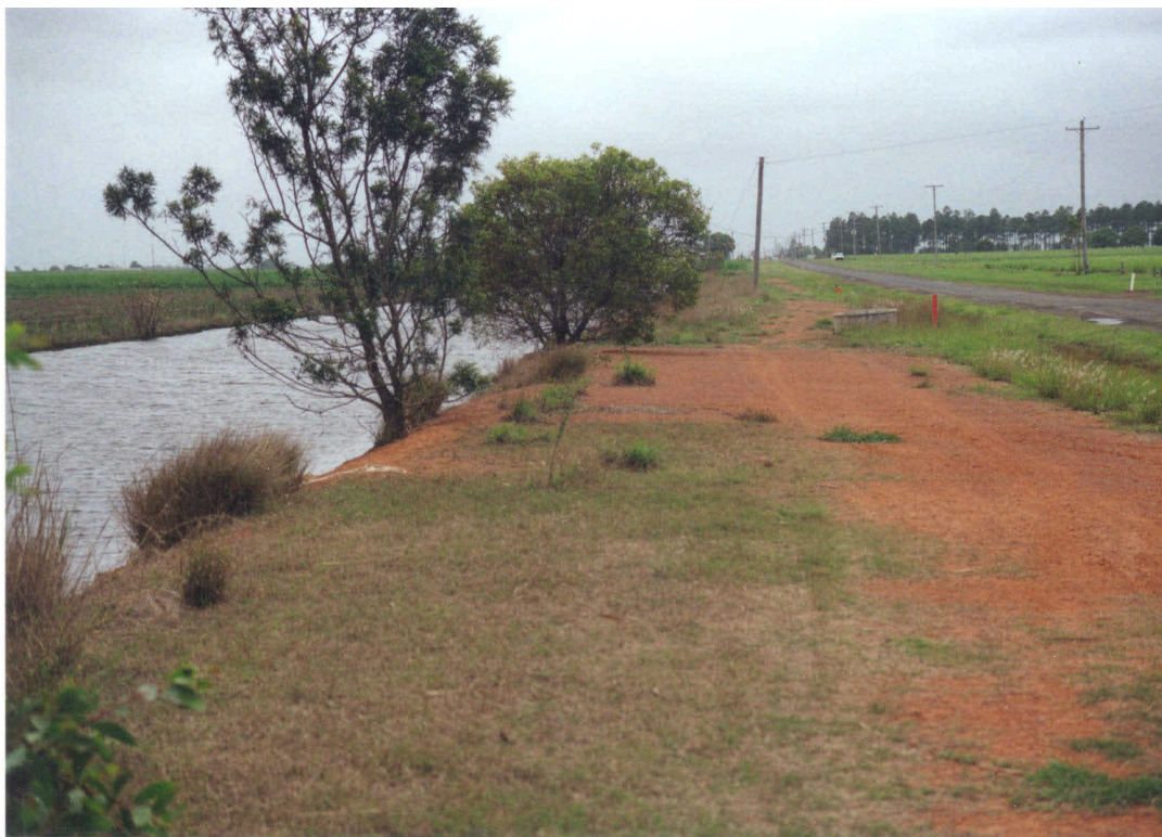
PHOTOGRAPH B-1 – ENCROACHMENT OF DAM ON ROAD RESERVE
