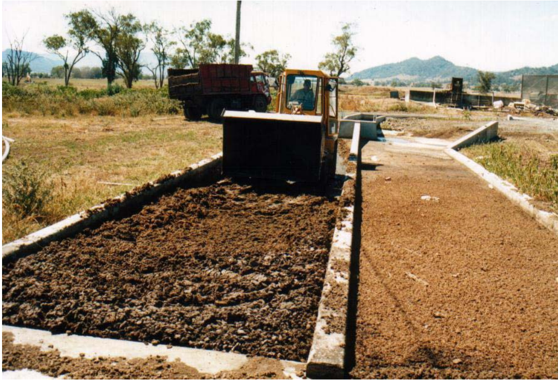
PHOTOGRAPH 1-1 - TRAFFICABLE SETTLING BASINS CURRENTLY USED FOR A 2400 SOW FACILITY
