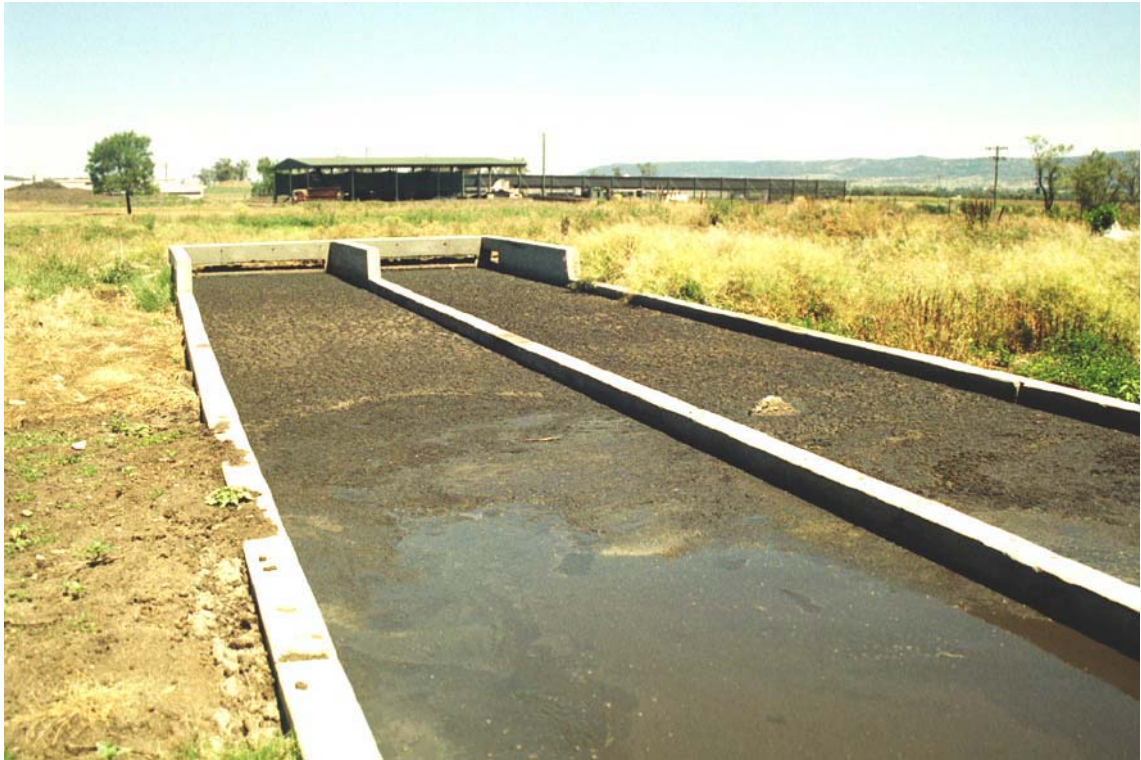
PHOTOGRAPH 1-3 - DUAL SETTLING BASINS (OVERLOADED)
