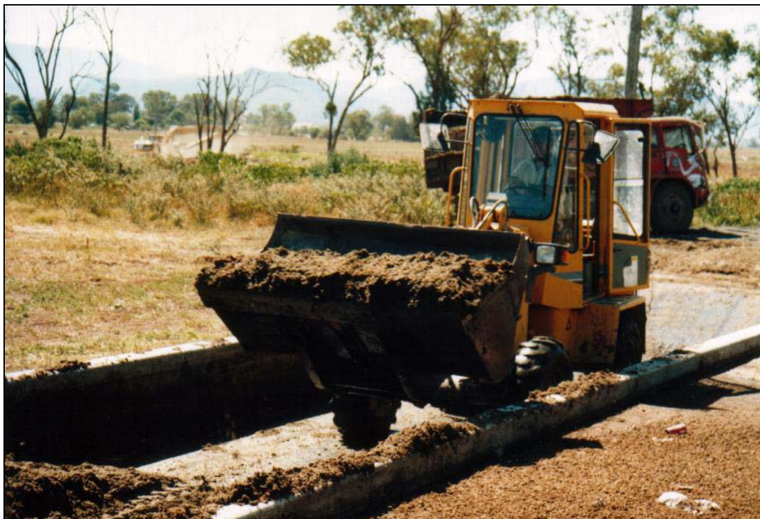
PHOTOGRAPH 1-2 - REMOVAL OF SOLIDS FROM SEDIMENT BASINS
